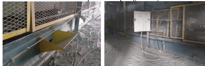
Gambar 5. Tampak luar spillage conveyor
