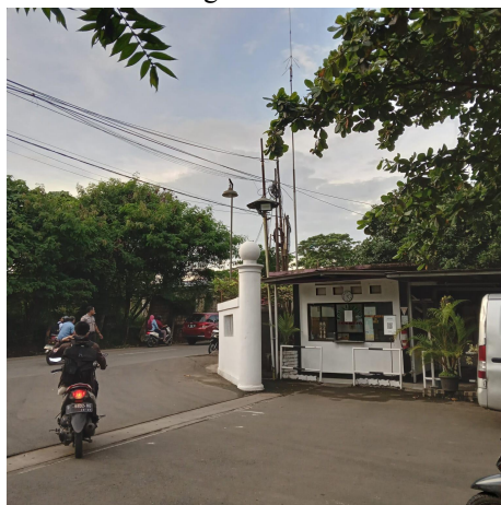
Gambar 2 Kondisi Pos Security
