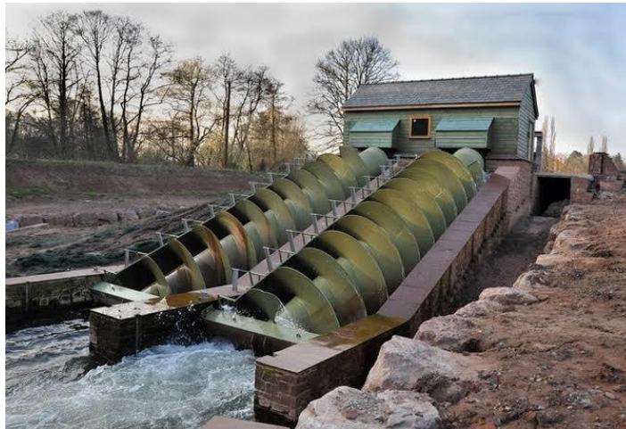
Gambar 3 Turbin Archimedes (sumber : https://www.hallidayshydropower.com/case-studies/ )
